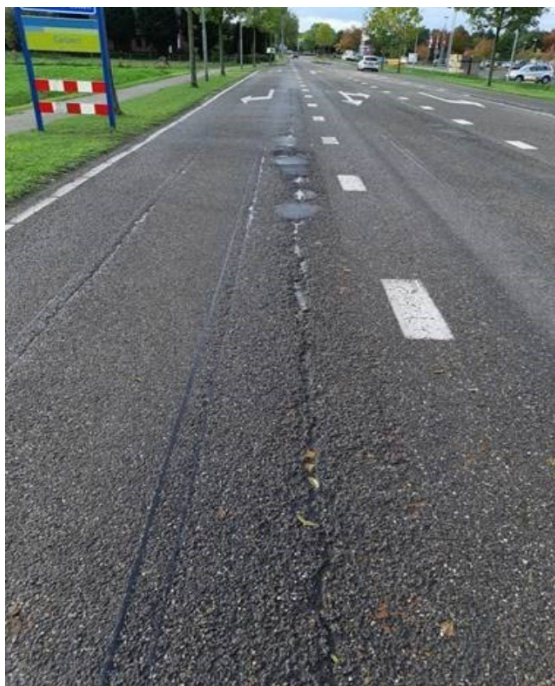
Rafeling/scheurvorming.
